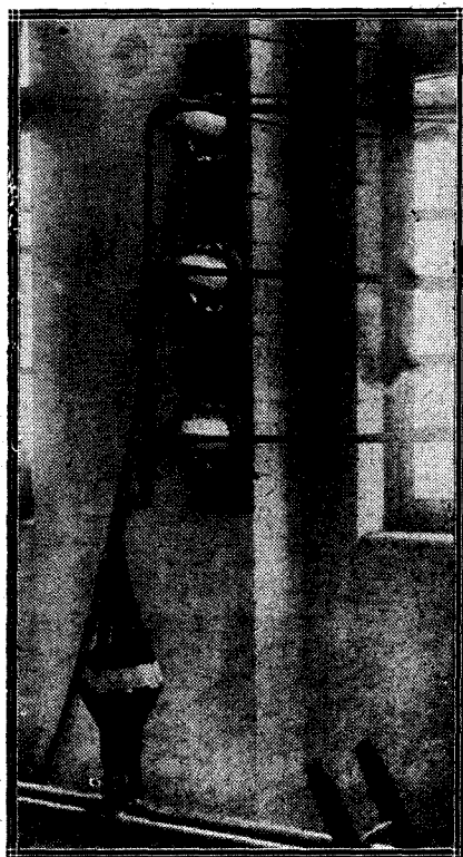
The earth connections at the Rugby station are no less carefully insulated than the aerial lead-in.
