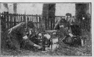
Another view of the engine and generator shown opposite, showing also the accumulator charging-board.
