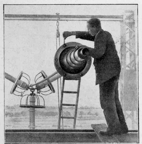
Adjusting the aerial lead-in and insulator at the Government wireless station at Hillmorton, near Rugby, claimed to be the world's largest wireless station.
