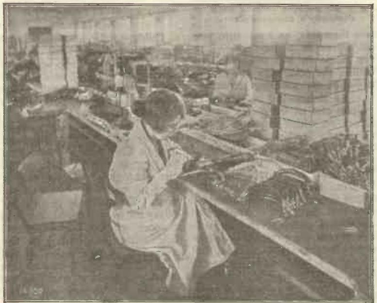
Assembling telephones at the B.T.H. works. Our photograph shows the closing of the clips on the leather head-bands.
