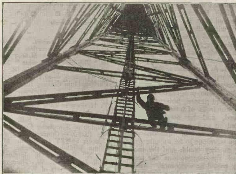
Our photograph shows a workman climbing up the inside of one of the masts at the Nauen Station. By holding the picture above the head and looking upwards, some idea of height is conveyed.
