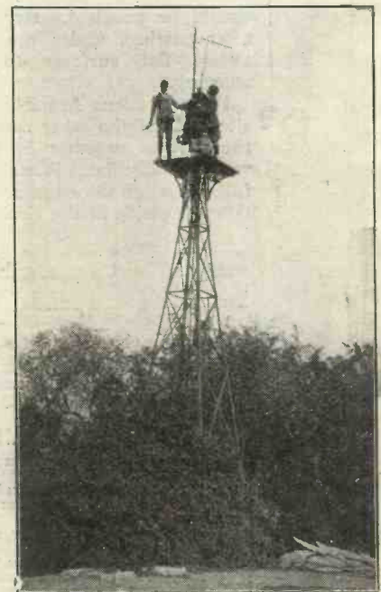
Employing a disused windmill as an aerial mast.
