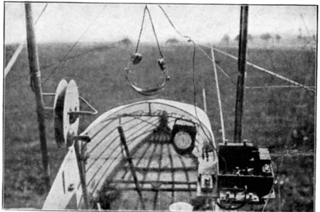
Fig. 3.—A Wireless Equipment on a Farman Biplane.
