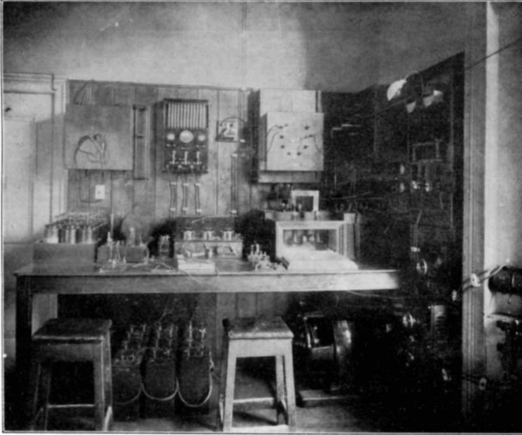
Portion of Instrument Room, showing Complete  $1\frac{1}{2}$ -K.W. Set and 10-in. Coil Transmitting Set.
