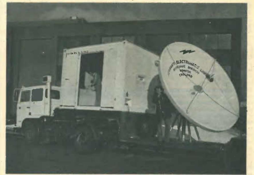
A transportable dish aerial, about 4m in diameter, is one of two supplied by Ferranti Electronics to British Telecom for use in trials for the business satellite.
