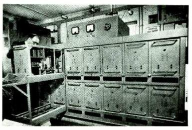
A section of the Wayne Kerr multiple-unit transmitter is shown withdrawn from its housing on the trolley provided for maintenance.
