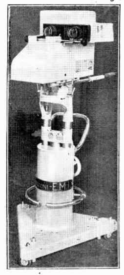
The latest model Emitron camera. The lens on the right of the picture is for focusing purposes.
