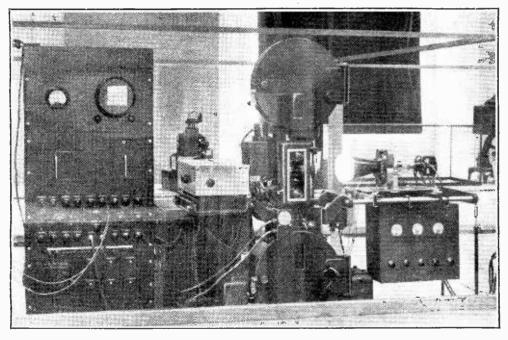
The Cossor film transmitter which is used to provide a signal for demonstrations when the Alexandra Palace is not operating.
