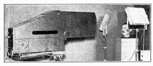
The Baird 30-line Spot-light scanner which was used in the B.B.C. transmissions up to 1932. The banks of photo-cells can be seen on either side of the head.
