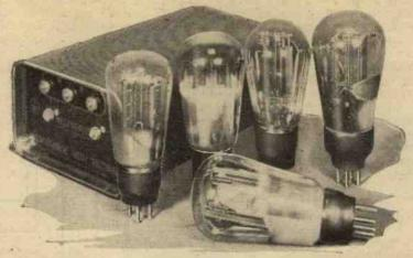
A Westinghouse metal rectifier is shown with a group of modern full-wave rectifier valves.
