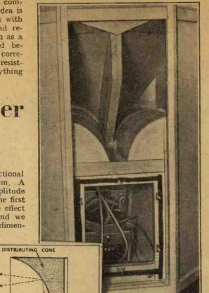
Front panels removed giving access to the giving access to the bass-chamber and twindiaphragm unit, and (left) diagrammatic section of cabinet, showing alternative sound paths.
