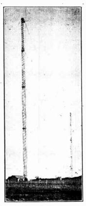
MASTS AT MOYDRUM. The aerial system of the new highpower broadcasting station of the Irish Free State. The transmitter has a power of 6okW. and was built by the Marconi Company.
