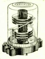
Colverdyne band-pass intermediate coil (Colvern).
