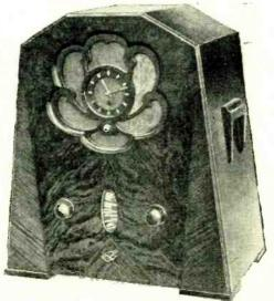
Ferranti 7-valve superheterodyne with station-scale and clock.
