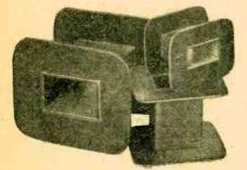
Savage's bakelite bobbins for transformer construction. Note the various sizes now available.
