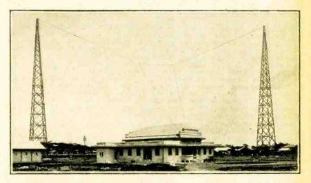
SHORT WAVES FROM SIAM. The Telefunken station at Bangkok. A double aerial is employed to permit of transmission on 14 and 17 metres without alteration to the tuning.
