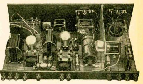
Rear view, showing H.F. transformers and mounting of H.F. valve supported on screen. Wave-changing switches are immediately over the tuning condensers.
