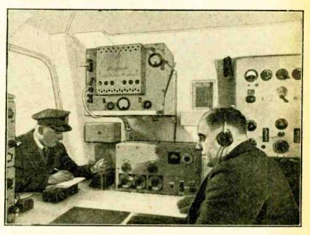
SHORT WAVES FROM THE AIR. The wireless cabin of the now famous "Graf Zeppelin." The New 50-watt short-wave transmitter is mounted above the other apparatus, while on the bench below is the short-wave receiver.
