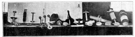
The photograph illustrates a number of aerial and lcad-in insulators. Those insulators which have a long leakage surface are generally the best.
