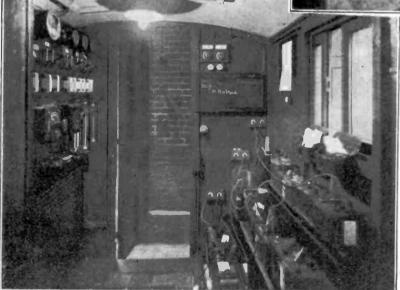
Above. — The motor generator and main switch - board at the charging station of The Park Motor Co., Ltd., in Wells Street, S.W.
