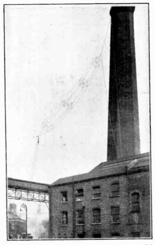
Fig. 1. The site of 5 WS, showing the aerial suspended from the chimney.
