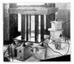
Fig. 9. The transmitting inductances and condensers.
