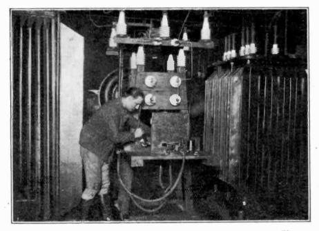
Fig. 4. The pneumatic relay, used for signalling in the high tension circuit. The are caused by breaking the circuit is extinguished by compressed air.
