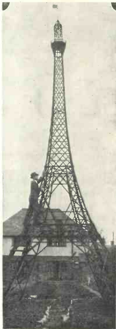
This aerial mast, which is a model of the Eiffel Tower, is 40 ft. high and has no guy wires. It was made by a young architect at Solihull, Warwickshire
