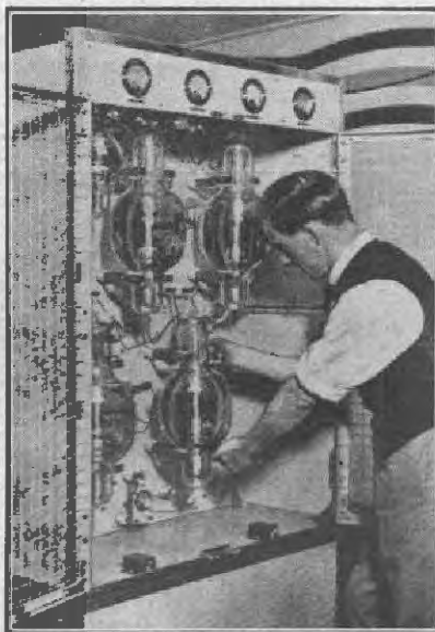
Putting the giant valves in the B.B.C. relay amplifier at Olympia. It fed about 400 loud speakers.
