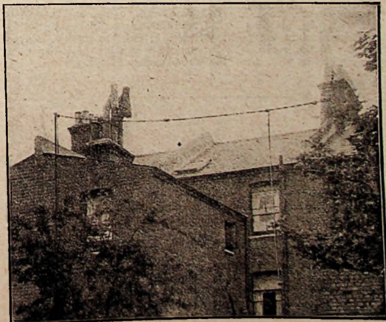
This aerial, having a long down-lead and short horizontal portion, gives excellent results.
