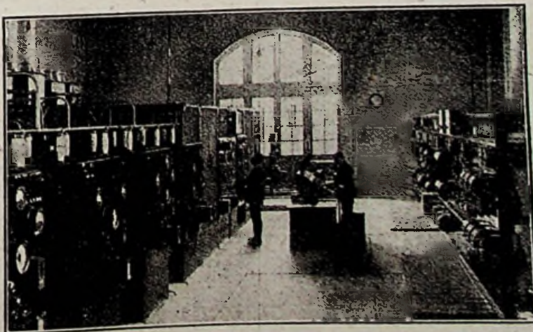
The valve room at Rugby, showing the power units, control tables and switchboard.
