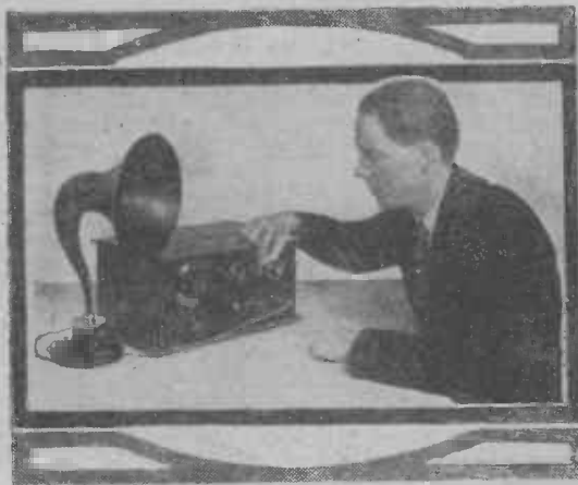
A loud-speaker set employing crystal or valve rectification as required
