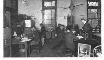
One corner of the operating room at Chatham. The telegraph instruments are connected to land lines to New York and Boaton for receipt and dispatch of radio messages to and from ships at sea
