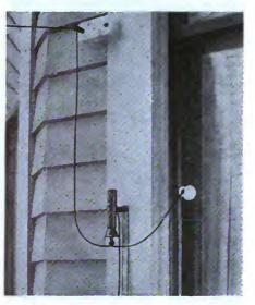
Figure 3-Effective lightning arrester installation
