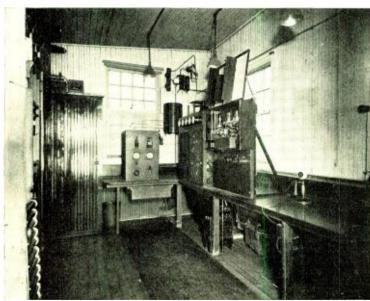
This photo shows the transmitting apparatus at the Radiophone Broadcasting Station KDKA at East Pittsburgh, Pa.
