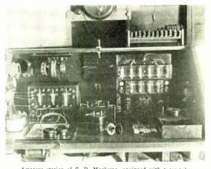
Amateur station of C. D. Macluran, equipped with a ten-tube transmitter and three-tube receiver
