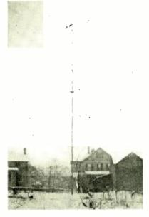
Antenna system of 20M station consists of six wires on 20 ft. spreaders, 35 ft. x 80 ft. above ground, total length 75 ft. natural period
