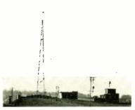
What WGY station looks like on the roof, showing one of the high towers and two-wire aerial
