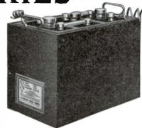
In the Westinghouse "B" battery you have a storage battery for "B" work-the latest development in radio practice. It has all the reliability and dependable performance of a storage battery and none of the disadvantages of a dry cell. The
