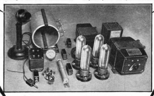
100 Watt Radio Telephone Transmitter
