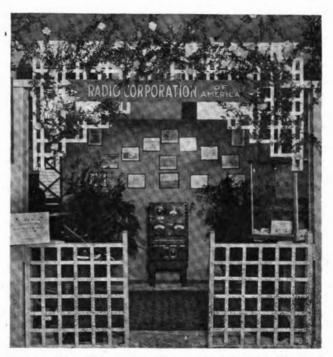
An interesting exhibit at the Radio Convention held in San Francisco. In the case at the right a Marconi coherer and a modern radiophone were exhibited showing the old and the new methods of radio reception. On a table behind the show case was shown a Marconi magnetic detector and an old-time tuner equipped with a crystal detector in striking contrast to the present day highly efficient vacuum tube receiver units
