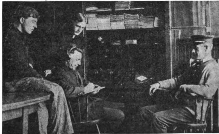
Modern fire fighting service requires the use of radio apparatus as evidenced by the installation at headquarters of the Cambridge, Mass., Fire Department
