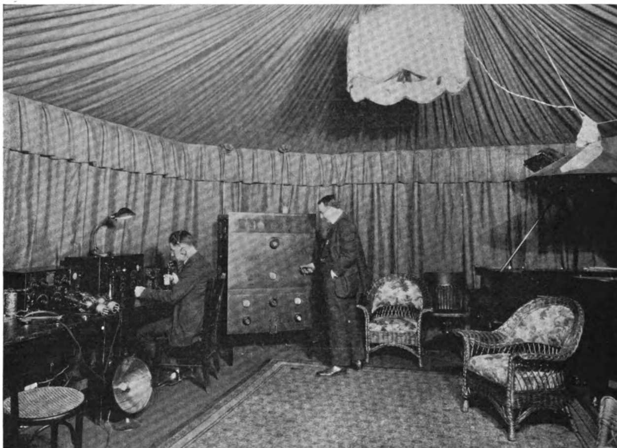
Studio of WDY Station. On the operating table at the left are located the receiving equipment of the station and all controls of the transmitting set
