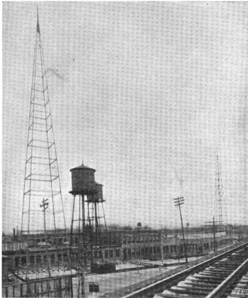
Towers and multiple tuned antenna at WDY Station, Roselle Park, New Jersey
