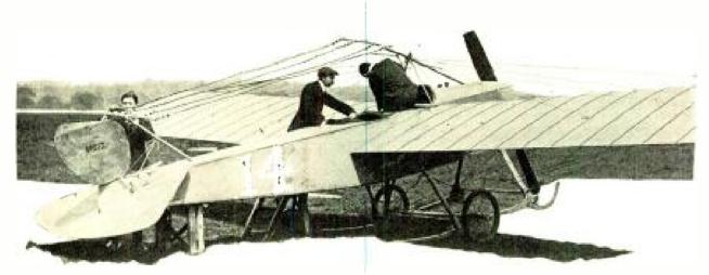
The successful wireless experiments by aeroplane carried out at Hendon. Mr. Valentine's Bristol monoplane is being fitted with the installation, only 40 feet of wire being necessary to complete the station on the aeroplane. The experiments proved successful
