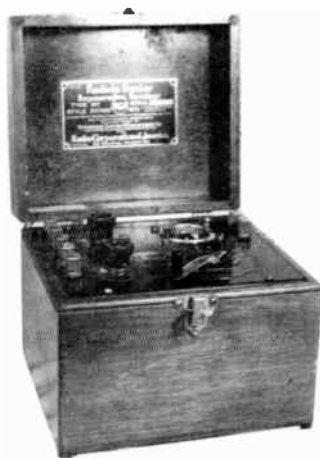
RADIOLA SENIOR TYPE RF REGEN. USES 199 TUBE MADE BY WESTINGHOUSE 1923 S.P. $65.00
