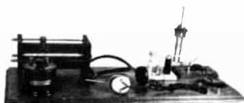
THREE SLIDE COIL RADIOELECTRON ELECTROLYTIC DETECTOR. WITH PLUNGER BATTERY.
