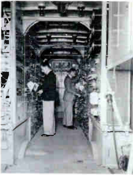
13d The first genuine Outside Broadcast. The Coronation, 12 May 1937. Interior of the Mobile Control van parked in Hyde Park. Note picture monitors head height at the far end
