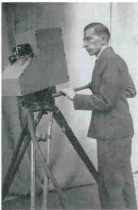
7a Bernard Greenhead with prototype Emitron camera. It had no viewfinder
