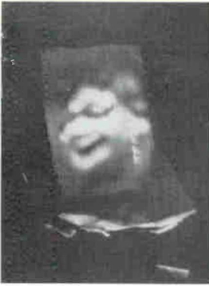
4a Thirty-line images photographed directly from the televisor. The picture of A.F. Birch, 1929 (right), shows a great improvement in definition compared with that of Stooky Bill, 1926
