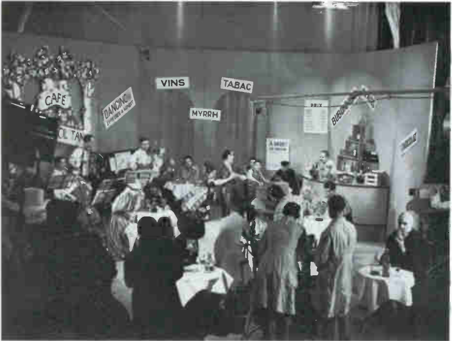
9d Café Cosmopolitan showing the three Emitron cameras, on left, on right and, mobile, in centre. The cameras are now fitted with viewfinders. Studio A, 11 February 1937
