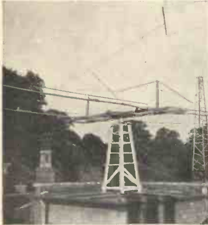
The rotary beam at G2FB.
