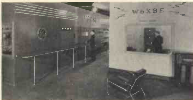
W6XBE which has been erected at Treasure Island, San Francisco, uses a 100 Kw amplifier and one of the new Alexanderson beam arrays. It is used to provide programmes for listeners in the Orient.
