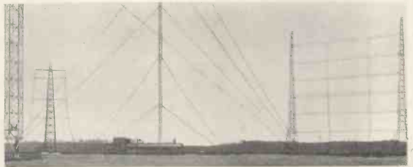
By the use of beam aerials of this type the German programmes can be directed to any part of the world ensuring good reception with only a low-power transmitter.
