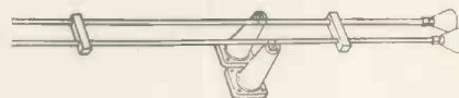
The feeders should be faced with ceramic insulators and wherever possible held in position by large stand-off insulators.
