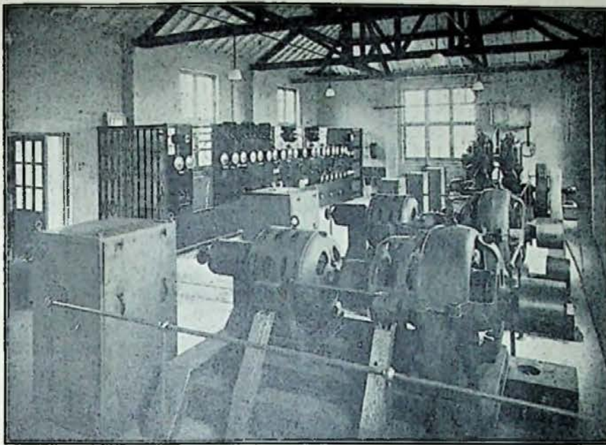
The Power Room at Northolt Wireless Station.
