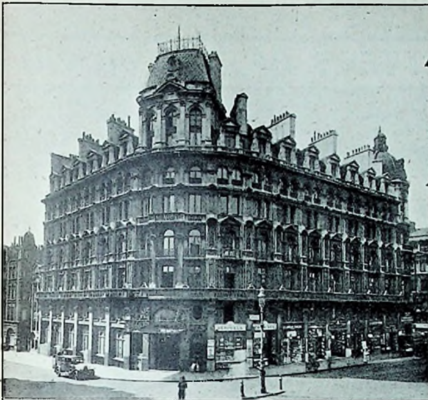
The Engineers' Club, Coventry Street, W., the Headquarters of the London Section of the Television Society.
