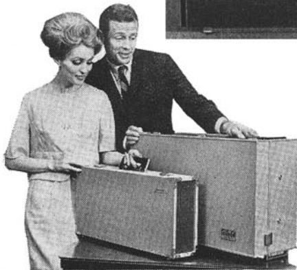
Above: Ampex VR303 fixed-head video recorder employing \frac{1}{2} in. tape. Left: Large and small cases containing Sony video recorder and camera kit.
