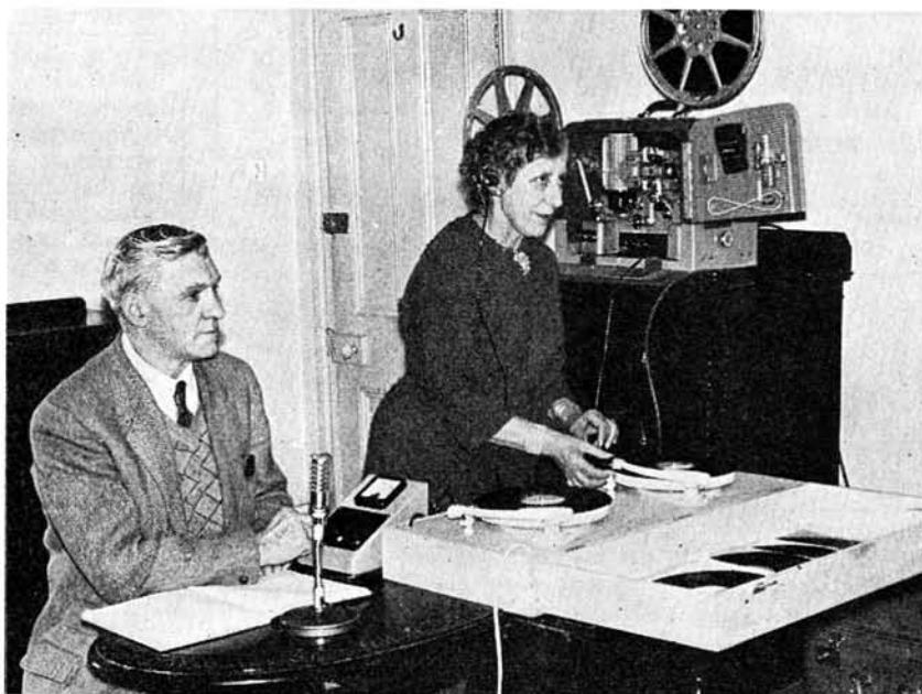
The Bell and Howell 640 is a fascinating machine for 16mm work. Equipped for optical and magnetic sound tracks, and supplied with plug-in magnetic heads, two supplementary sound tracks can be laid down on Zonal stripe, after the first has been recorded.
