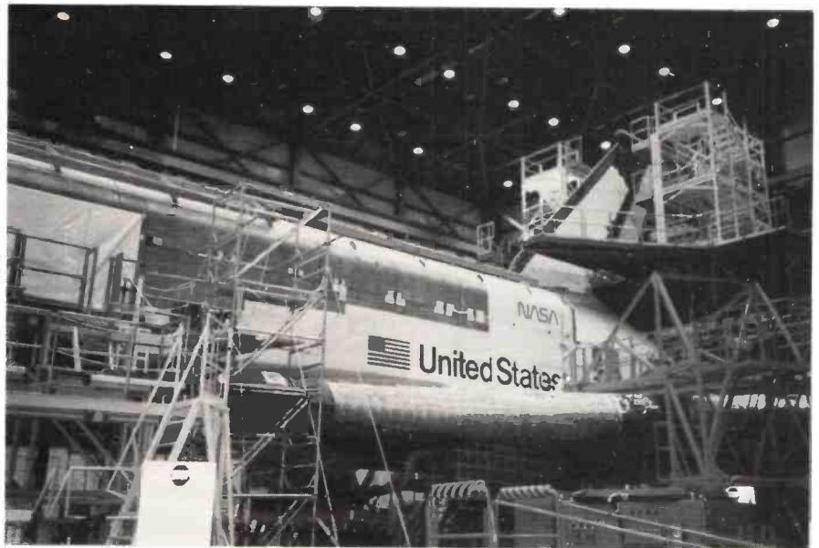
Behind all the scaffolding and covers, Columbia is readied for her next mission which will be in 1989.
