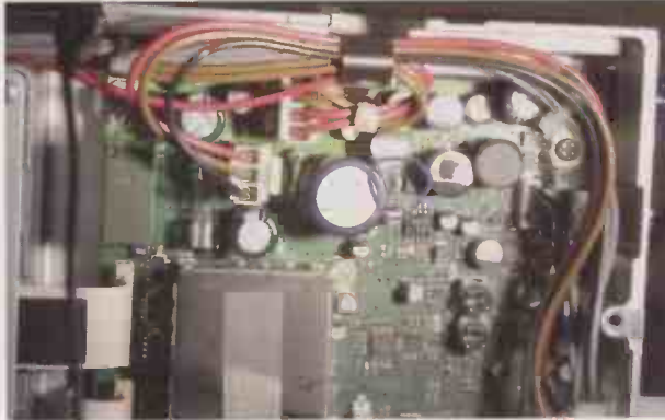
● The coupling capacitor to be removed.
