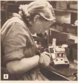
6. The next operator adds the gang condenser and the intermediate frequency transformer, soldering a small number of additional components and wires, all furthering the circuit to completion
