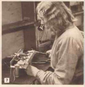
7. At this state the chassis has progressed considerably, as you can see. The volume control, wave-change switch and scale plate have all been added, together with other small condensers
