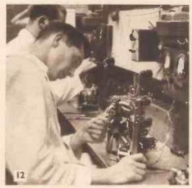
12. The Radio Frequency circuits are tested and the trimmers of the R.F. coils adjusted, which is then checked at pre-determined points on the scale
