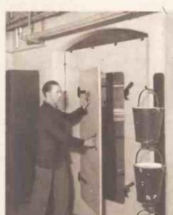
The brick walls at the base are over four feet thick. The basement of the B.B.C. is practically bomb-proof. The Gas-proofing Co., called in to discuss how the whole of the B.B.C. corridors (over a mile long) could be made gas-proof, stated that it would be an eight-weeks job. Gas-proof doors are being fitted in the basement, so that by the time the job is finished two whole floors will be quite gas-proof.
