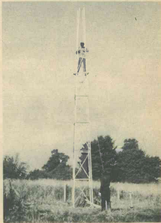
The Heathkit Aerial Tower in process of erection
