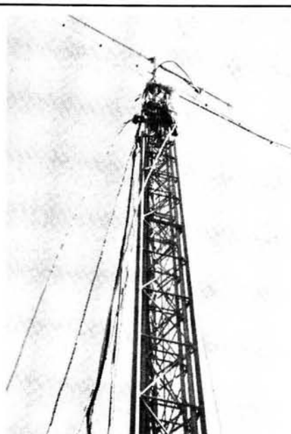
Antenna inspection at GM4CAA/P on Lowther Hill
