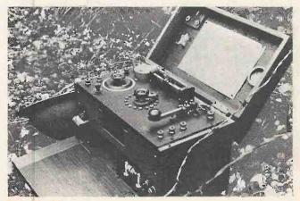
Fig. 1: 50 watt Trench set made by the Marconi Company
