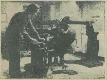
In this equipment the standard cine film is projected direct into the television camera. The film is used as a fill-in in broadcast plays, etc. Trainee Mrs. Dorothy Jones is operating the apparatus.
