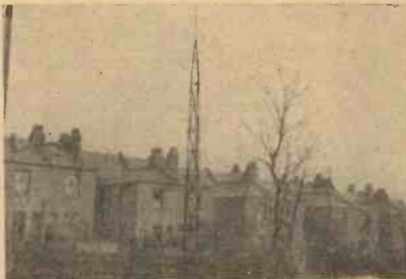
Fig. 1.—The lattice mast built by the author of this article, and which was blown down in the recent gale.
