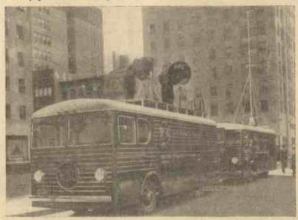
America's first mobile television station, delivered recently to the National Broadcasting Company at Radio City, New York. One van provides operating positions on the roof for the cameras, and the other a "trolley" aerial for relaying the pictures back to Radio City.
