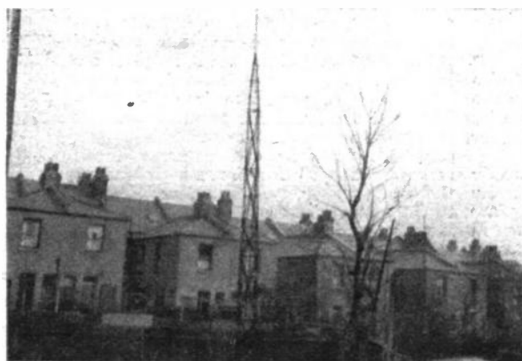
A lattice mast built by the author of this article, and which will be described in next week's issue.
