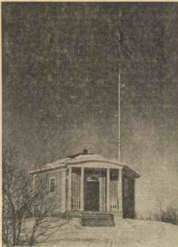
This little building at Kiruna, Lapland, represents Sweden's most northern wireless station.
