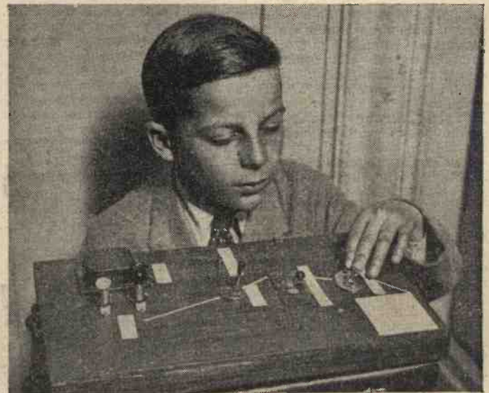
KENNETH CHEESEMAN, with his invention for stopping would-be car thieves. It is operated by a hidden electric switch which, immediately the car thief puts his foot on the accelerator or takes off the brake, causes an electric siren to shriek, illuminates a flashing red light in the headlamps, and thus attracts the attention of police and passers by.
