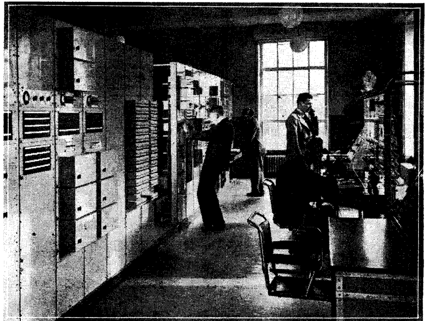
The Control Room of the new Broadcasting House, Glasgow.
