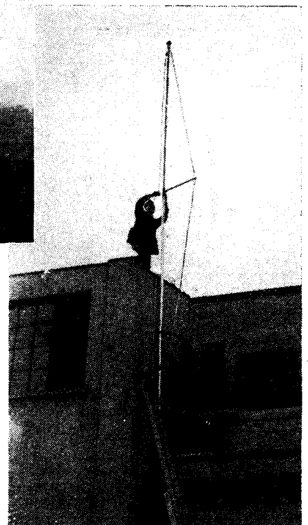
The upper mast being fixed in position on the lower.
